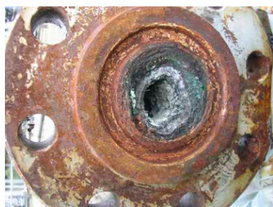
Figure 4: Scale build up within a pipe ( 8 \mu\text{Sv/h} dose rate at pipe exterior). Picture courtesy of ExxonMobil
